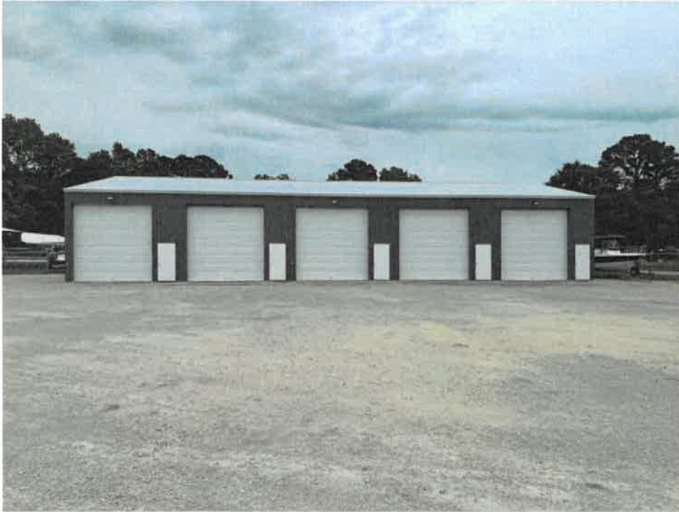
Image #3) Example front elevation of building #6 (50x100). Note: This is NOT the proposed color scheme. See proposed color scheme in Attachment D.
